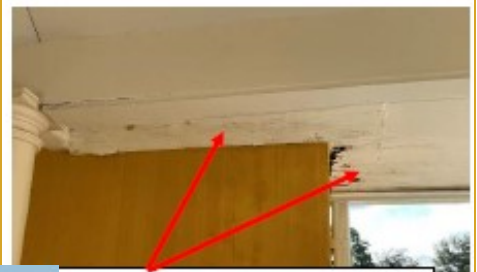
We observed signs of water/moisture on the soffit under the tile roof system on the East side.
